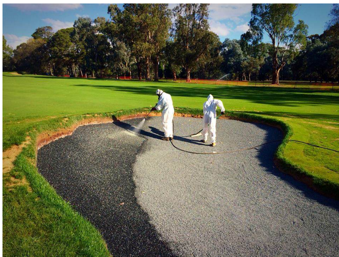
Figure 2: Installing the polymer on a Kustom Bind bunker
