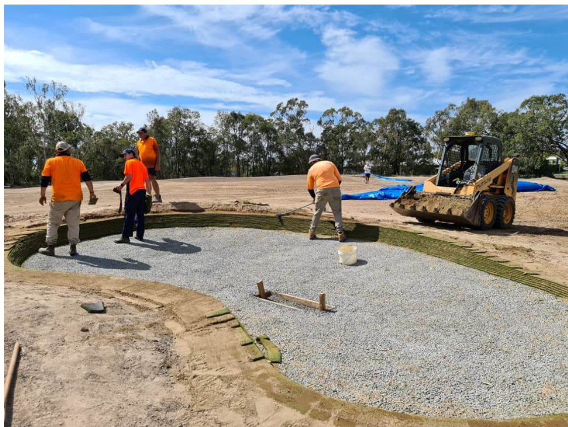
Figure 1: Constructing a Capillary Bunker with Eco Bunker faces
